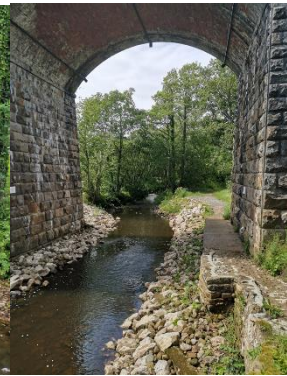
Under the viaduct
