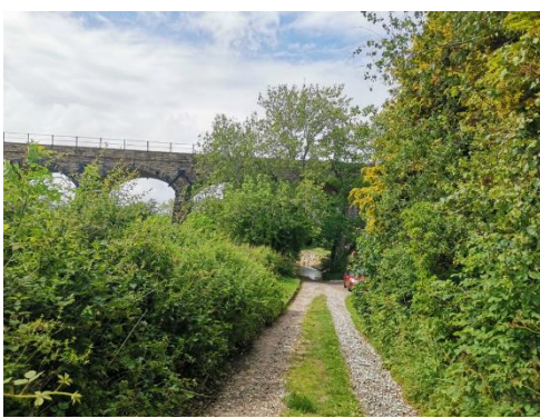
Towards the viaduct
