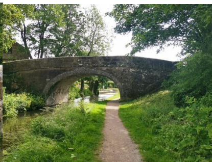
Under this bridge
